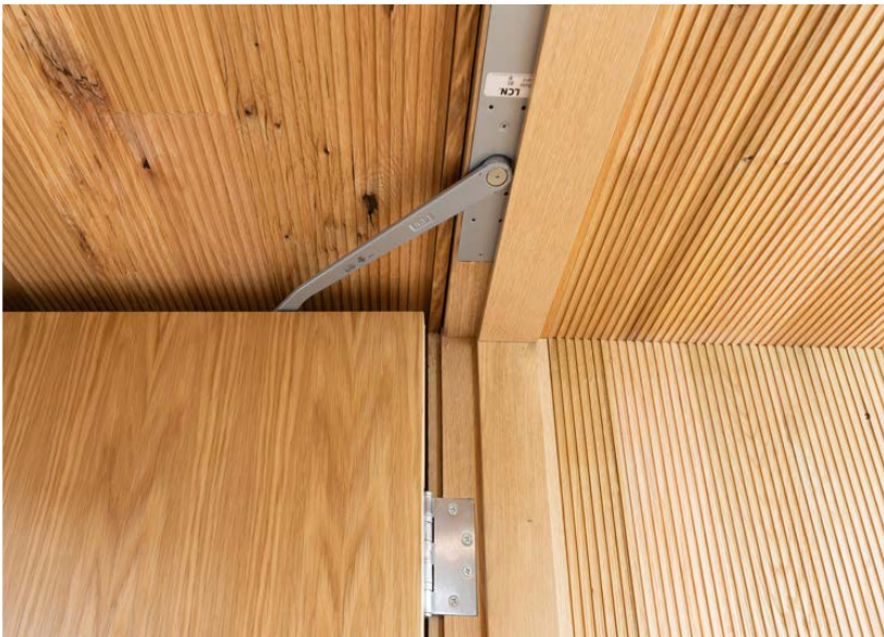
Left: Traditional Surface Mounted Overhead Closer; Right: Concealed closer hidden within wood door frame
